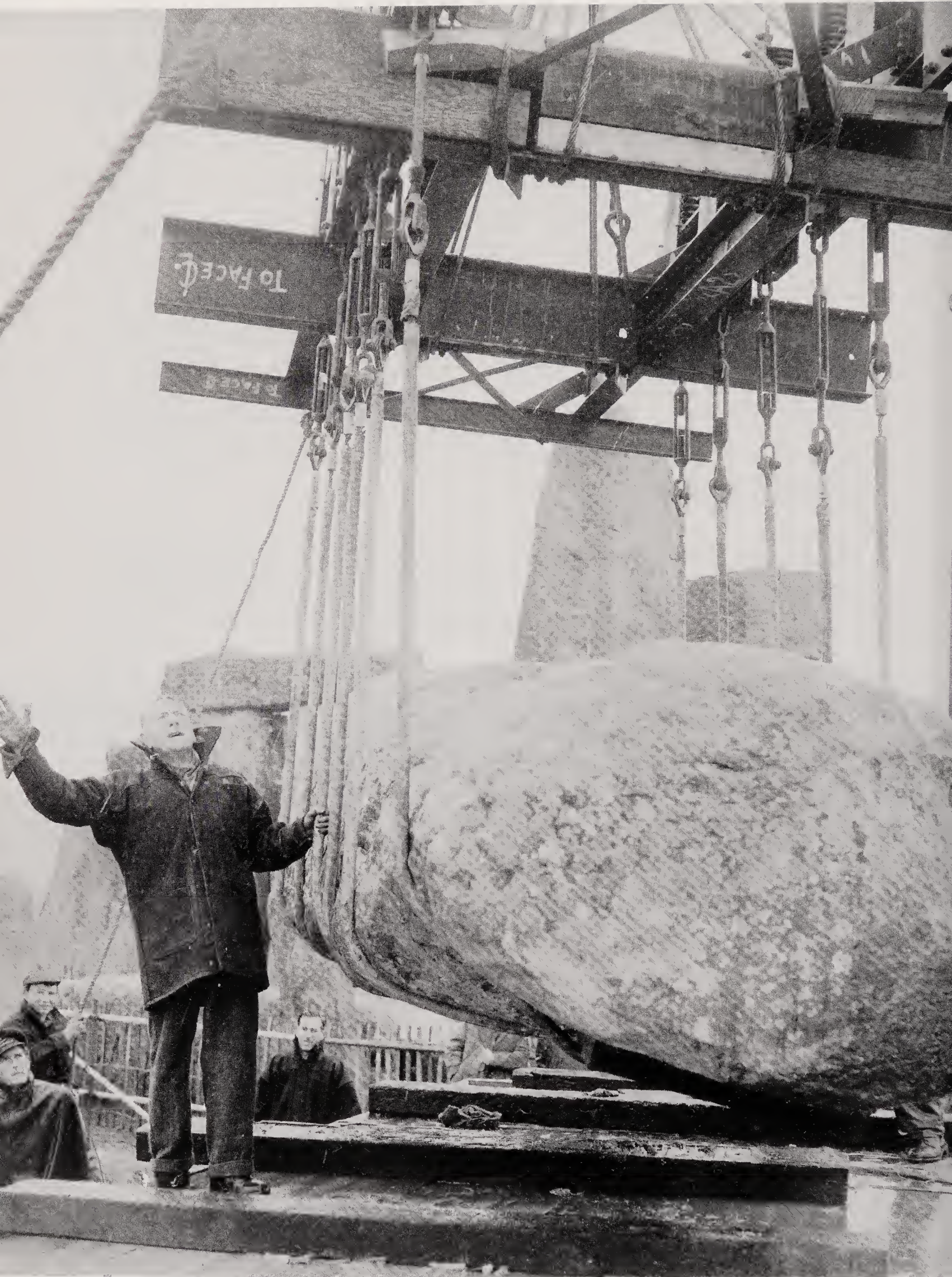
In 1958 a crane was used to lift one of the eighteen-ton lintels of a fallen trilithon back into place as part of a restoration project.
