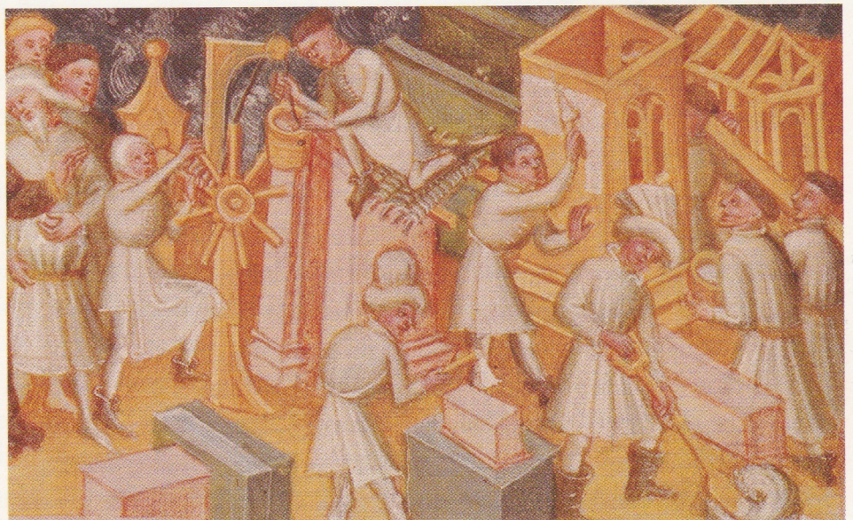
Masons at work, shaping stones, mixing mortar and hoisting it up in buckets.
